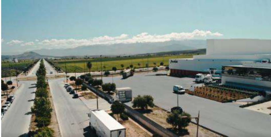
FIGURE 9 PROFITEGRA INDUSTRIAL PARK
