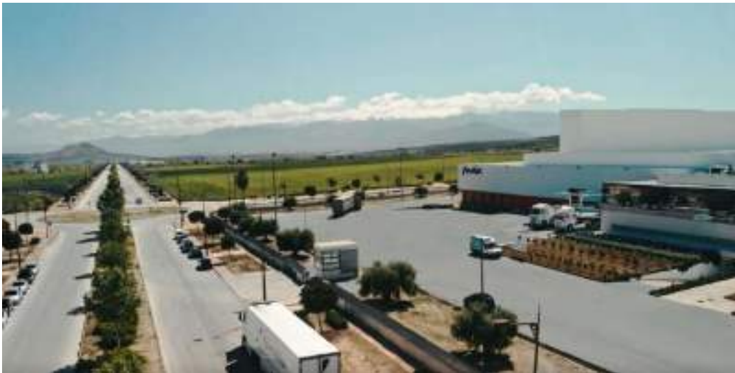
FIGURE 4-2: PROFITEGRA INDUSTRIAL PARK (2)
