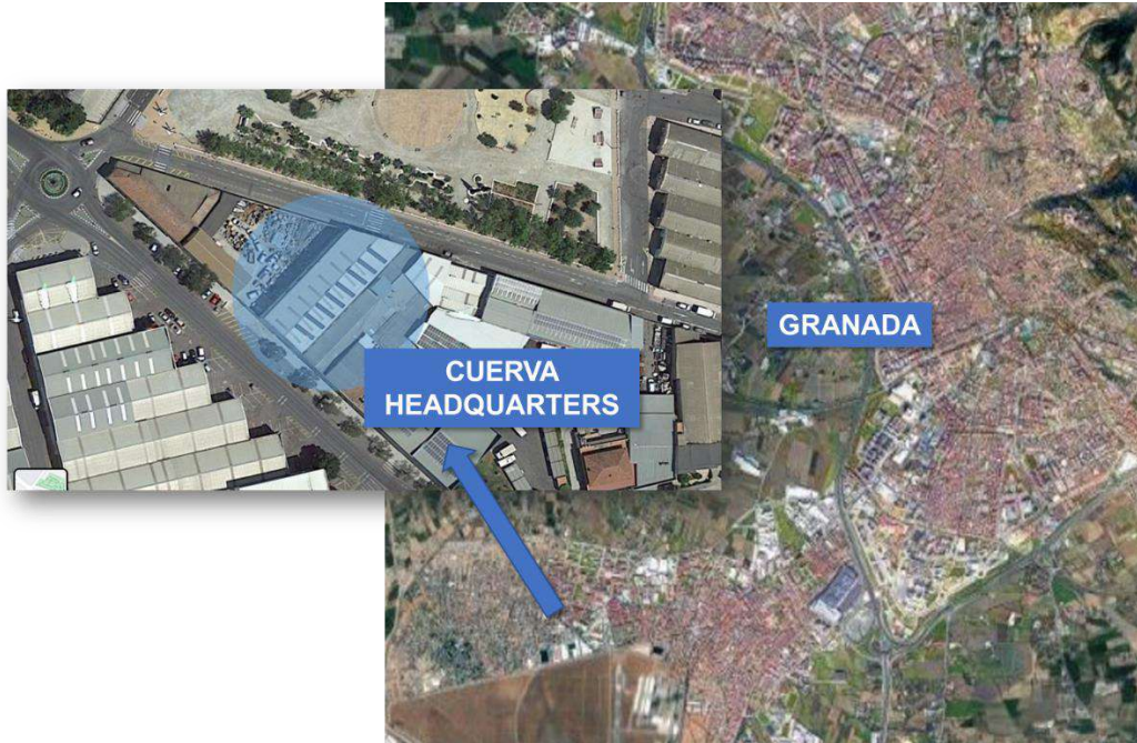
FIGURE 4-5: THE CUERVA HEADQUARTERS LOCATION
