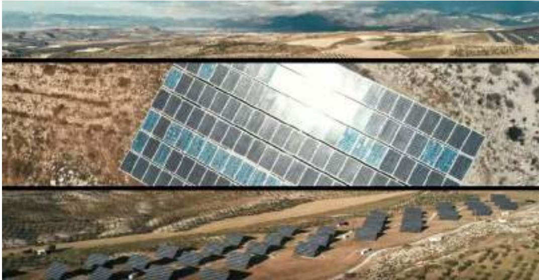
FIGURE 4-3: PROFITEGRA INDUSTRIAL PARK (3)
