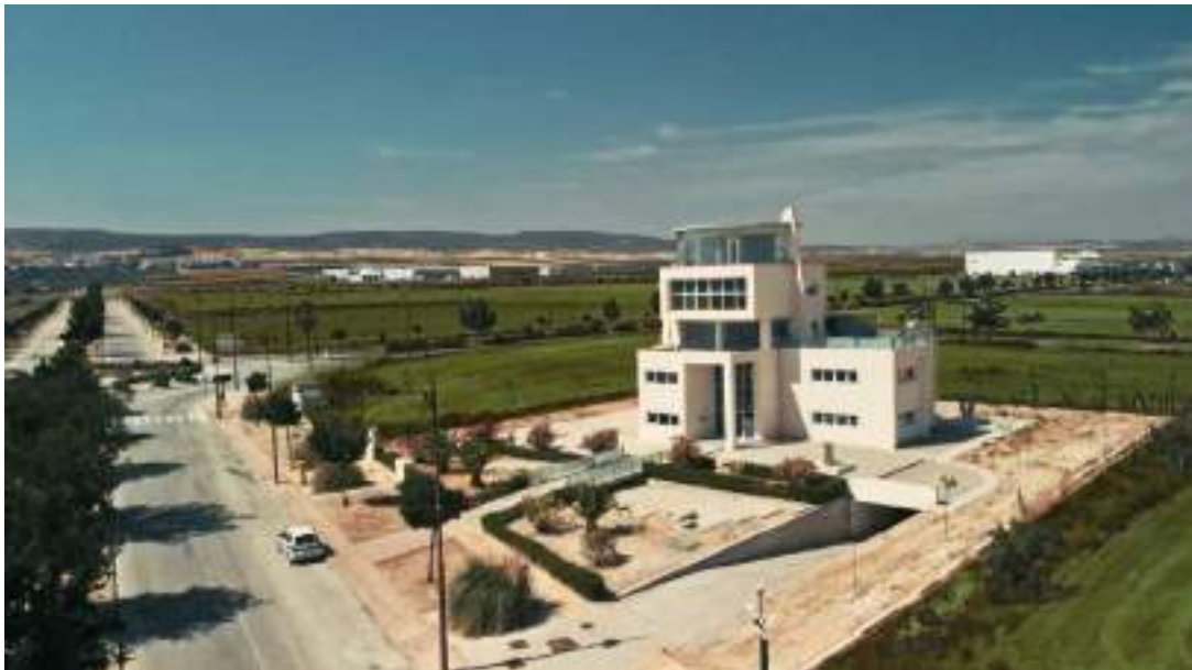
FIGURE 4-4: PROFITEGRA INDUSTRIAL PARK (4)
